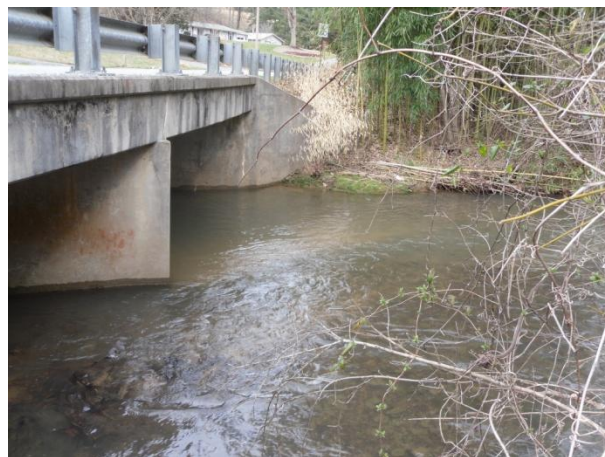
Figure 1. Site 2 – Bob Peoples Bridge on Sinking Creek Road
